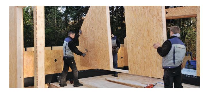
EGGER OSB4 is a synthetic resin bonded flat pressed board with a three layer structure consisting of (micro Veneer) specially thin aligned stands of up to 160 mm which ensures the panels are not only strong but have high load bearing characteristics enabling larger panel sizes of up to 6 m.
