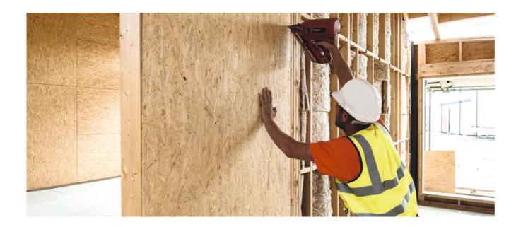
EGGER OSB3 panels are produced on state of the art continuous production lines, where we optimise the strand orientation and moisture levels of the panels. This means that the panels are not only strong, offering high load bearing capacities but reduce possible dimensional movement due to atmospheric conditions.
